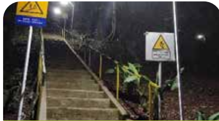
Penambahan penerangan Addition of Lighting
