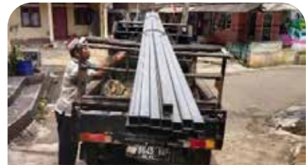
Pengangkutan material dan alat Transporting material and Equipment
