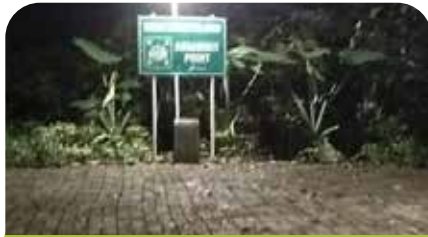
Penerangan Assembly Point Assembly Point Lighting
